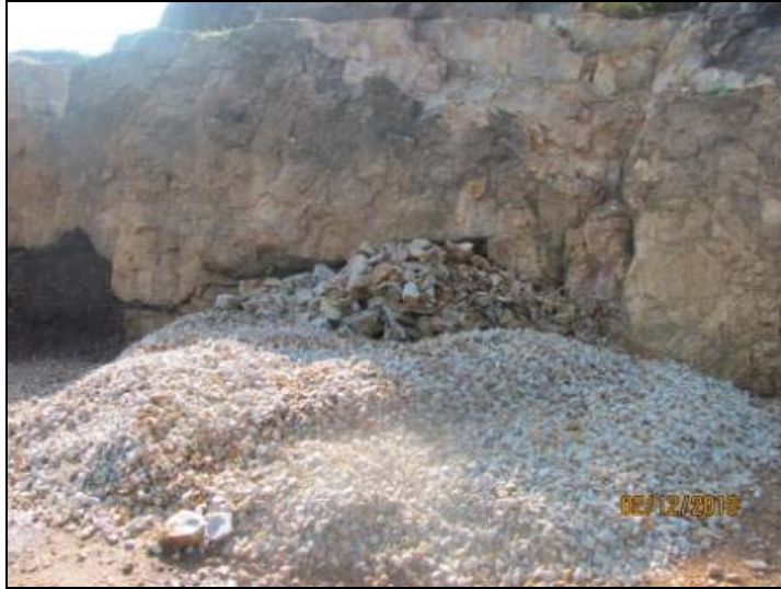
Photo showing one location of Mende Quarry site
