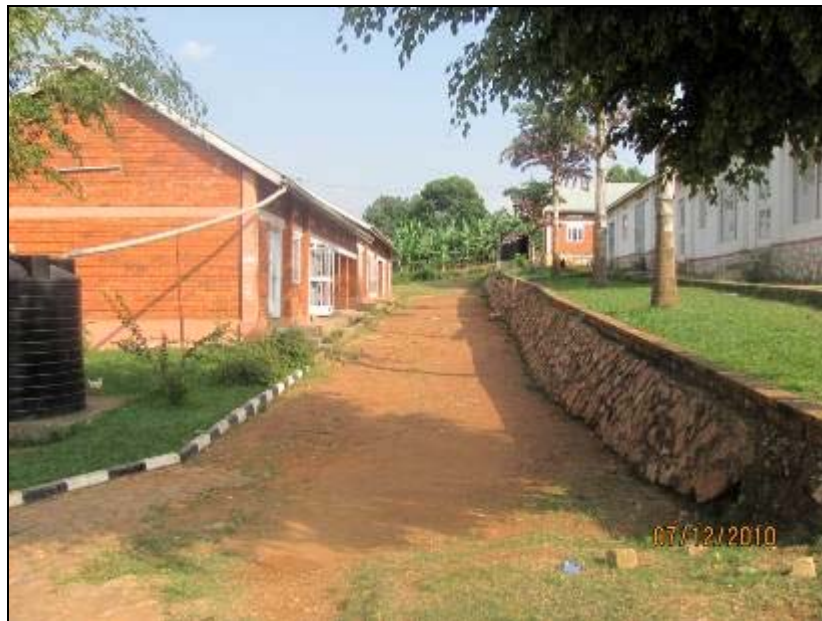
Photo showing the newly completed Vocational Block III\\
