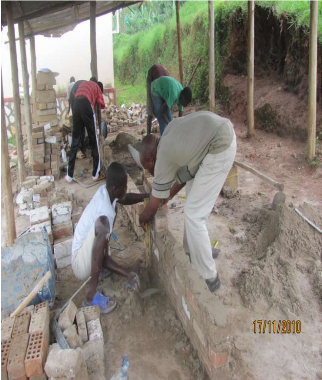
Brick laying instructor at one of the training sessions
